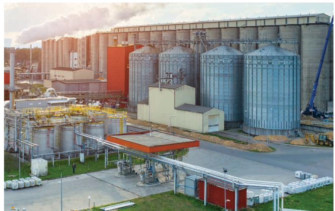
Grain Processing Facilities
