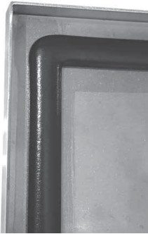
Polyurethane poured-in-place door gasket
