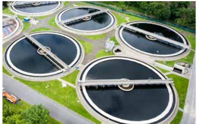
Waste and Wastewater Treatment Facilities
